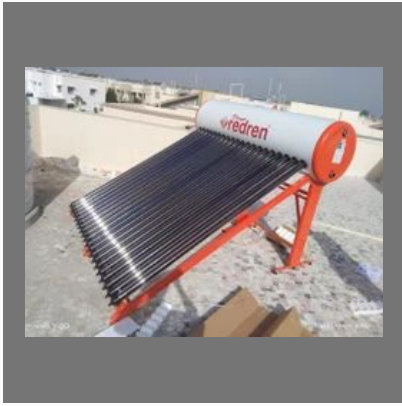
Solar Water Heater
